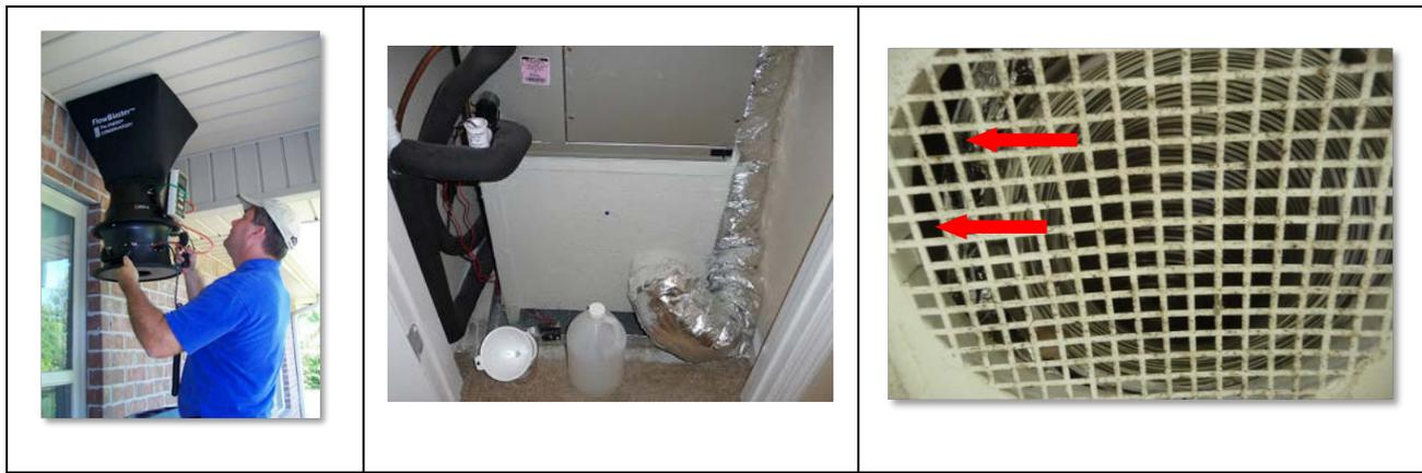
Figure 1. Study findings included: a) airflows often fell short of design values, b) outdoor air duct with hard kinked turn at plenum as shown, c) outdoor air intake duct disconnected from grille collar, resulting in over 40% of the “outdoor air” coming from the attic/soffit area.
