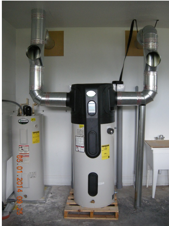
Figure 5. Ducting of intake and exhaust air using an 8-in. smooth metal duct.
