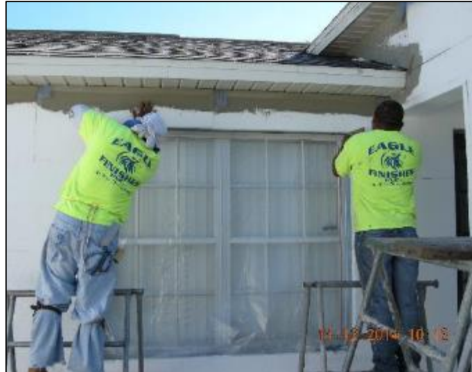
With no change in exterior finish color, the building has similarly low solar absorptance pre- and post-retrofit.
