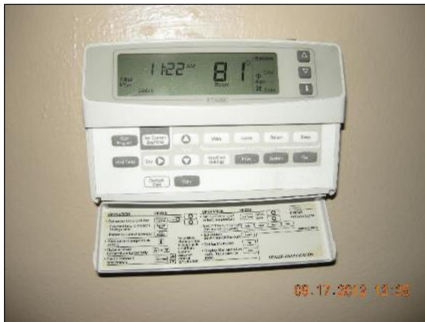
Figure 38: Site 28 existing thermostat, a Trane XT500C programmable model
