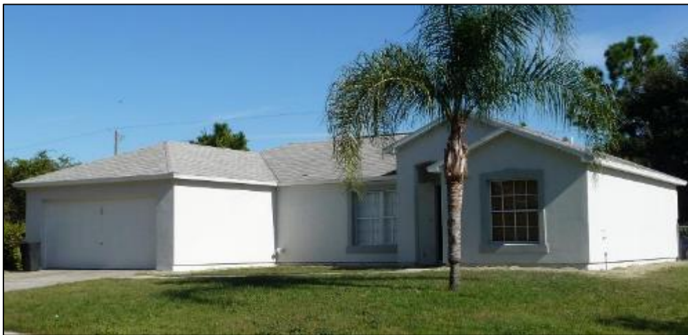
Figure 14. Site 54 attachment of 2-inch polystyrene insulation (top left), final textured coat application (top right), completed exterior insulation finish system retrofit (bottom)
