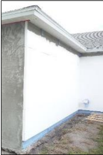
With no change in exterior finish color, the building has similarly low solar absorptance pre- and post-retrofit.
