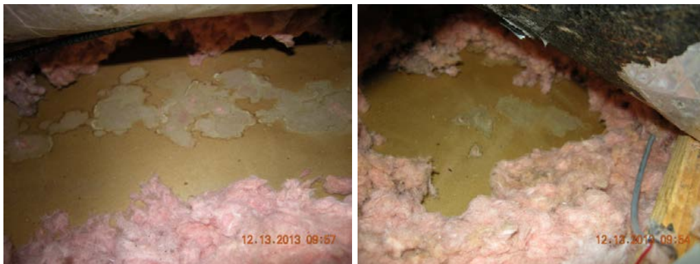
Figure 137. Historical moisture issues in attic under ductwork
