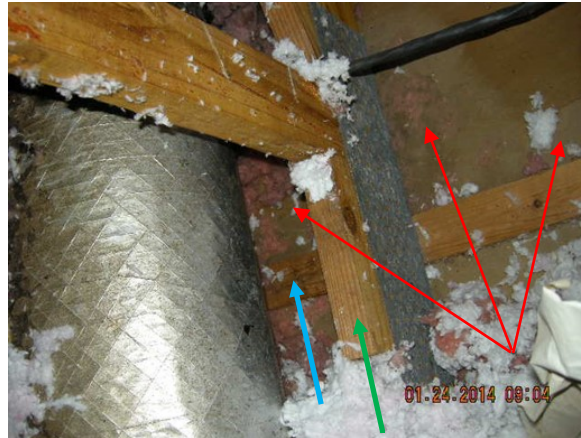
Figure 139. Past water stains observed in ceiling drywall directly above living room
