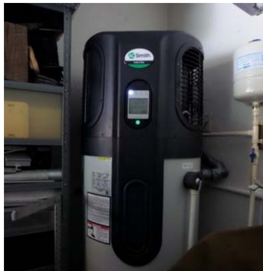
Figure 150. HPWH retrofit existing conditions
