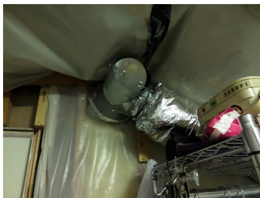
Figure 142. Second-floor closet with shared supply ducting and open damper
