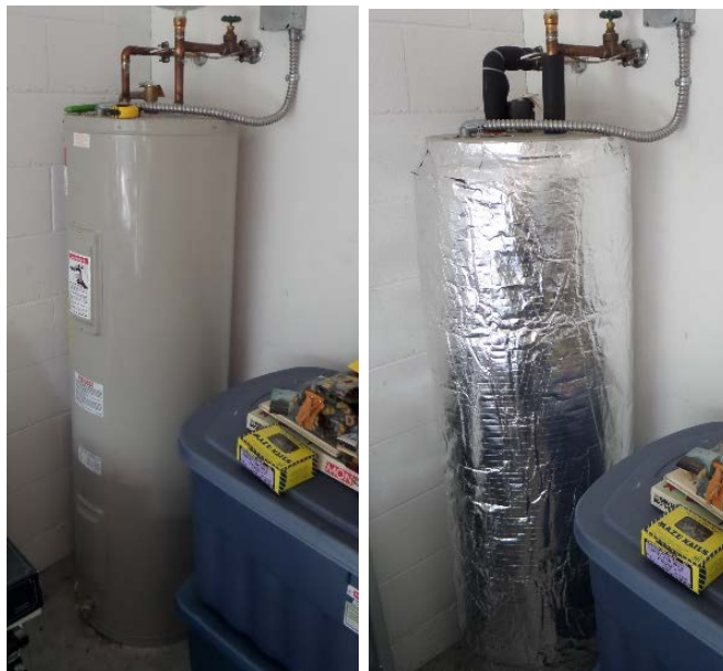
Figure 11. Site 54: Uninsulated tank and hot water pipes (left); insulated tank (R-3.5) and hot water pipes (R-3)
