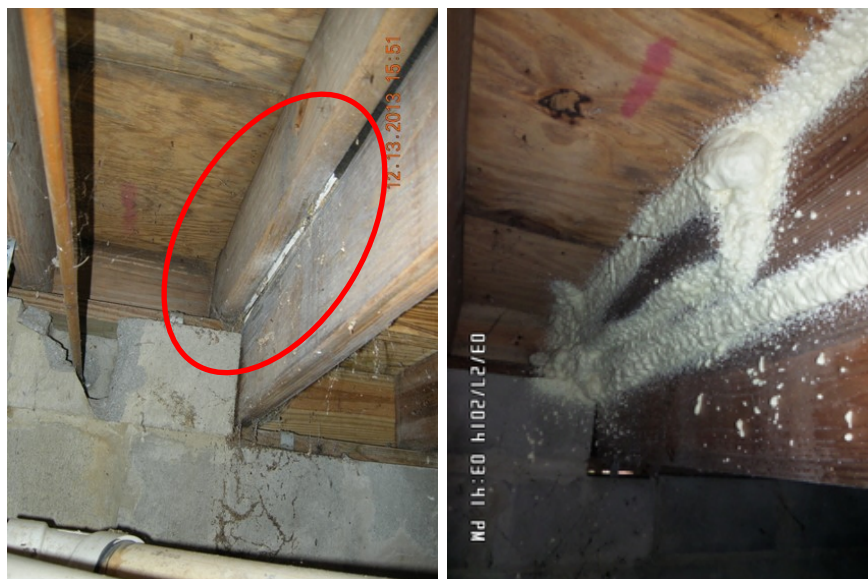
Figure 147. Crawl space floor transition areas unsealed (left) and sealed (right)
