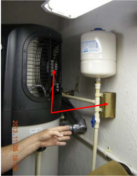
Figure 148. Site 19 HPWH initial installation (left) and noise attenuation retrofit (right)
