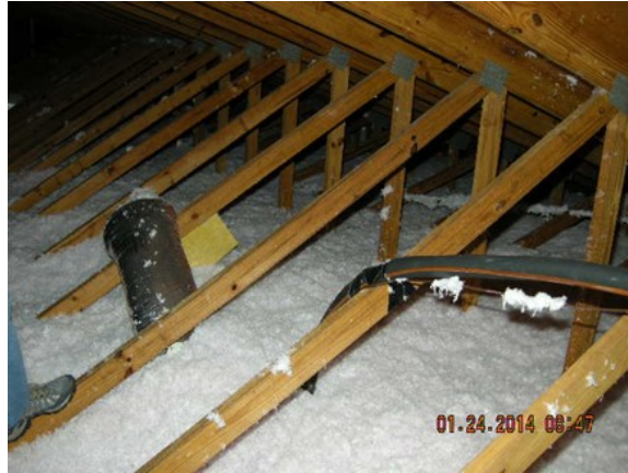
Figure 136. Buried ductwork
