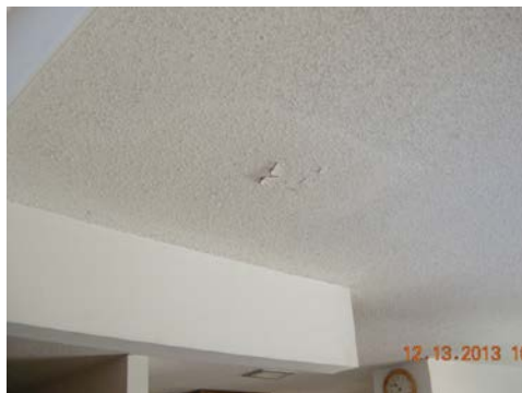
Figure 138. Ceiling damage close to room's supply duct
