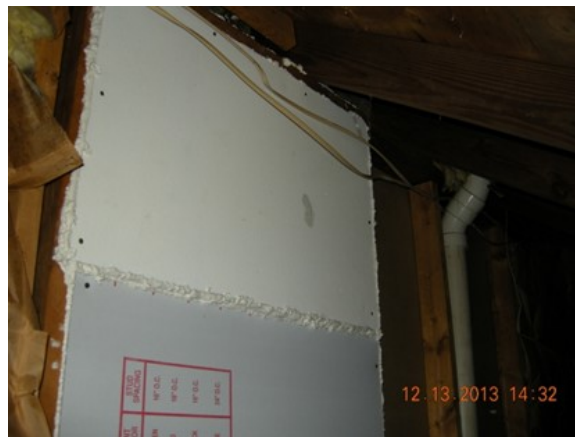
Figure 145. Air barrier installed
