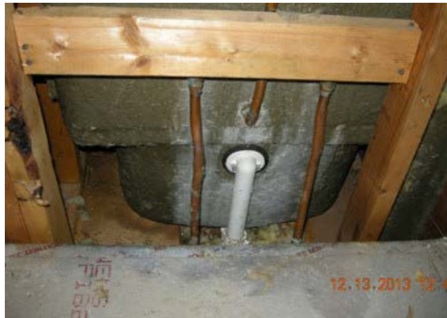
Figure 143. Missing air barrier behind tub
