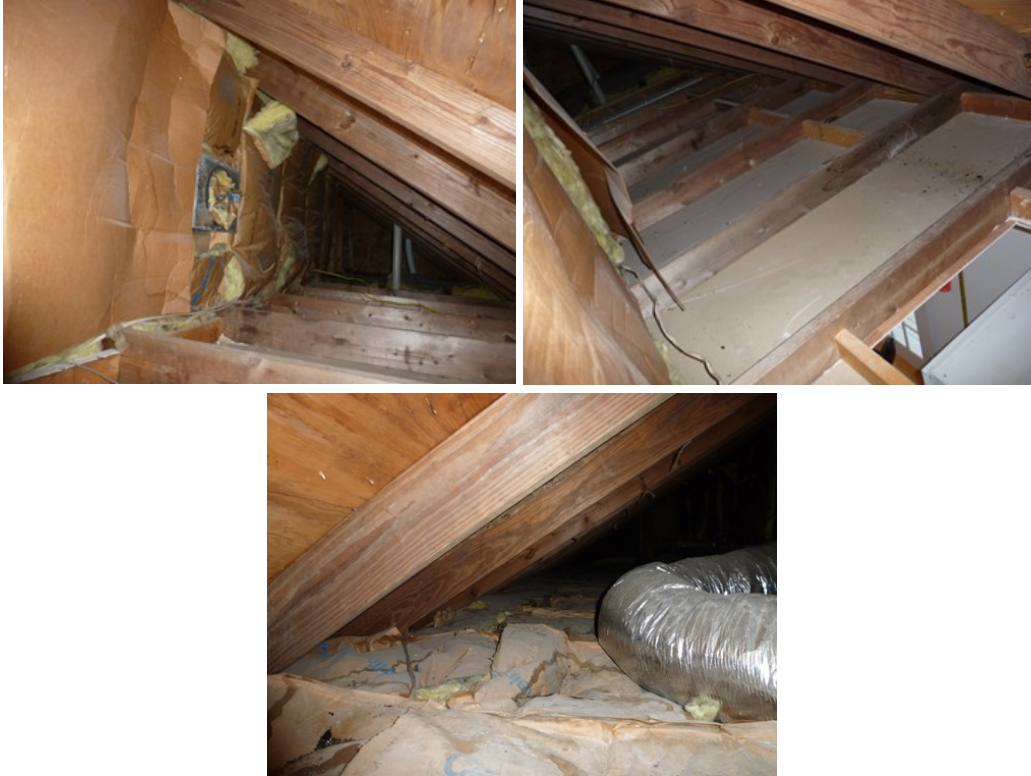
Figure 146. (a) Attic knee wall exposed kraft (top left), (b) knee wall with cardboard covering exposed insulation (top right), and (c) batt insulation with kraft paper exposed (bottom)
