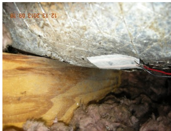
Figure 140. Moisture sensor strip adhered to bottom of ductwork
