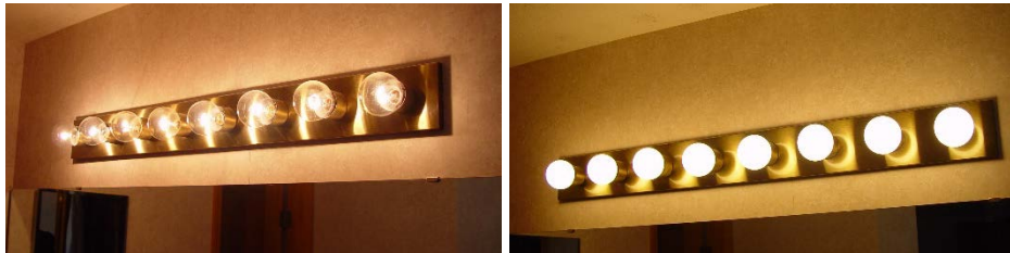
Figure 14. Site 7: Eight-bulb retrofit from 360 watts of incandescent bulbs (left) to 72 watts of CFLs (right)
