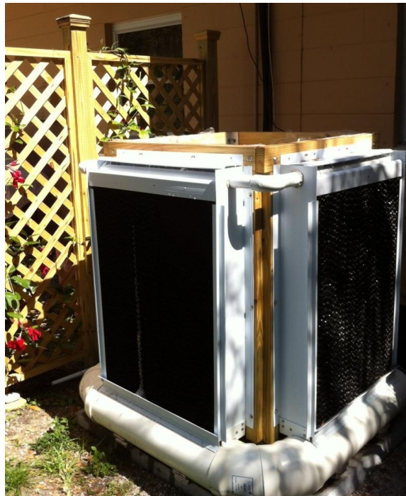
Figure 19. Field Installed Phase II prototype
