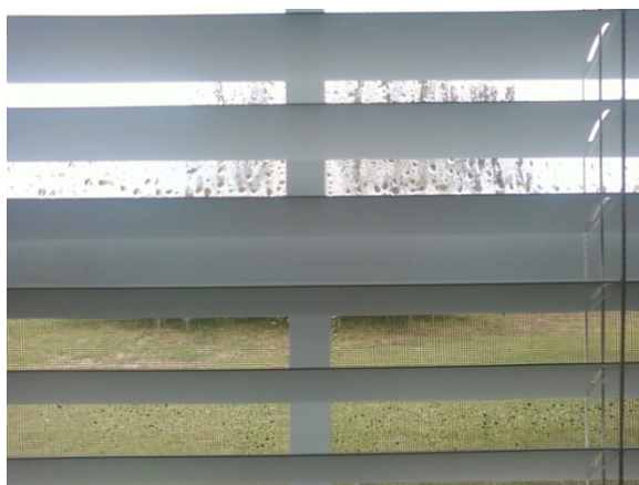
Figure 13. There appeared to be more condensation on the glass portion than on the screened portion of each tight home window
