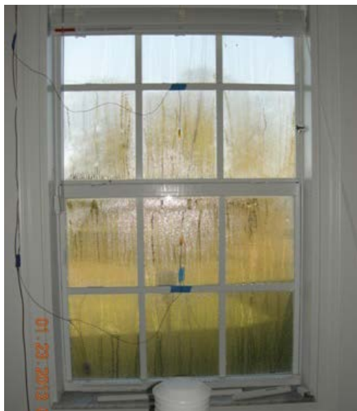
Figure 24. Unvented tight house north-facing window condensation January 23, 2013
