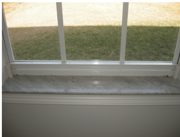
Figure 4. Windows are shimmed to allow leakage
