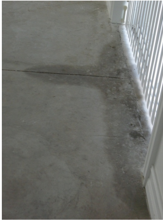
Figure 15. Tight home condensation residue by sliding glass doors
