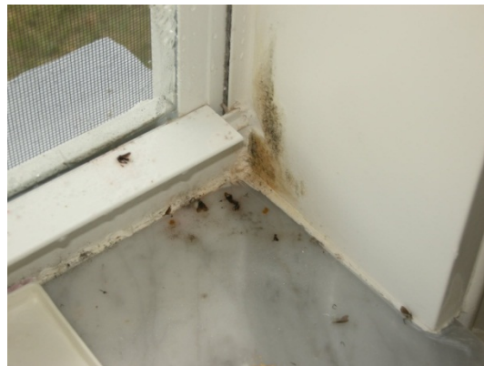
Figure 16. Mold surrounding a tight home window
