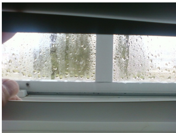
Figure 14. Considerable condensation accumulated
