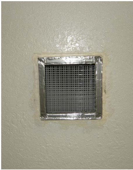
Figure 2. Ceiling penetration for planned leakage
