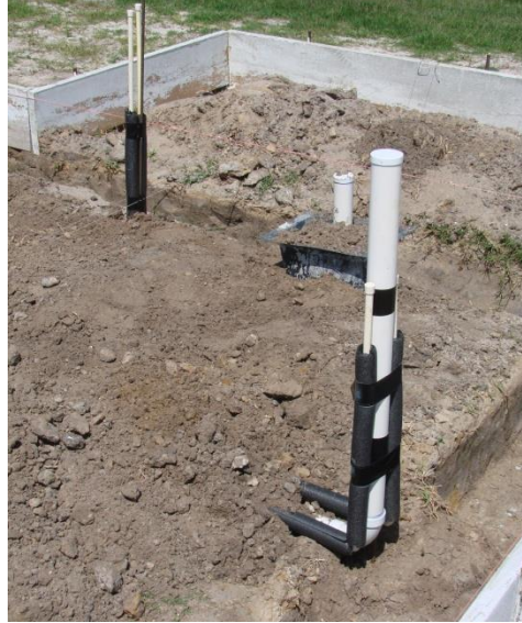
Figure 4. Insulated pipes under the slab foundation.
