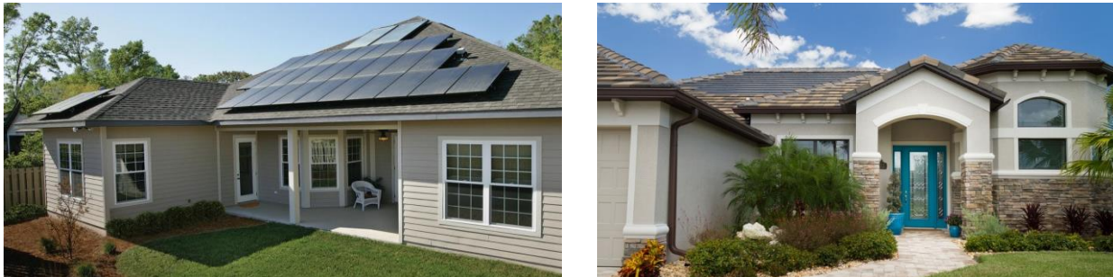
Figure 116. TWH (left photo) and LSH (right photo) have each been successful at standardizing ZNER designs, and offer ZNE homes as an option.
