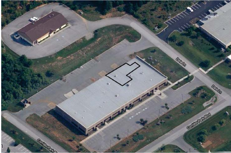
Figure 6-1 VRF Field Site 1 – EPRI Lab, Building 2, Knoxville, Tennessee
