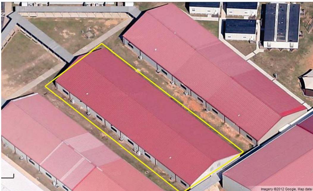
Figure 6-7 VRF Field Site 2 –Faith Academy, Mobile, Alabama
