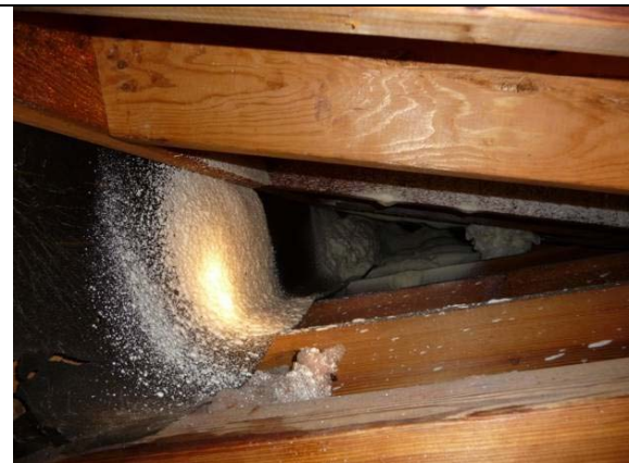
Figure 13 Beginning of north side sealing. (LaHiff)
