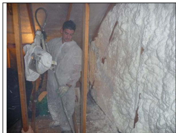
Figure 9 Technician finishes up kneewall and floor cavity insulation/air tightening. (Photo credit Ian LaHiff)
