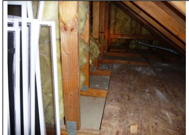
Figure 1 View of kneewall and main floor space (far), and bonus room wall and floor cavity (left).
