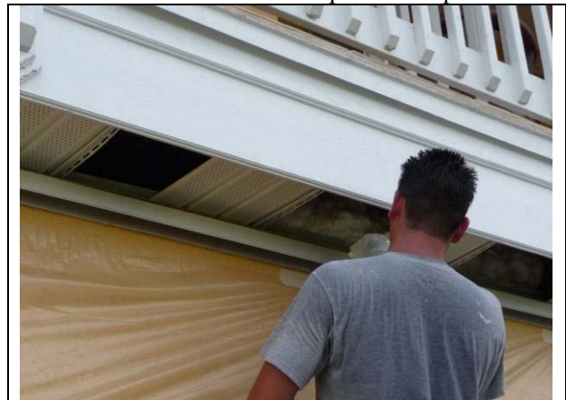
Figure 6 Foam application into west soffit area. (Withers)
