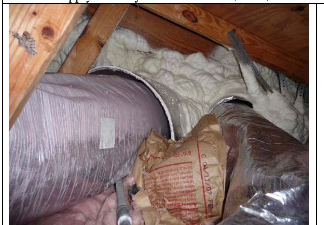
Figure 5 East side floor cavity isolated from the garage attic; a protective vapor barrier/thermal barrier sleeve isolates the foam from the exterior of the supply ducts to reduce the condensation potential. (Withers)
