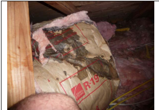
Figure 4 Moisture condensed on flex ducts and accumulated on insulation materials placed in contact with the supply ducts by the homeowner. (Withers)
