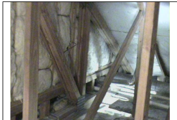
Figure 8 Photo of IR image above. The floor cavity at the bottom of the wall is open to garage attic. (Withers)
