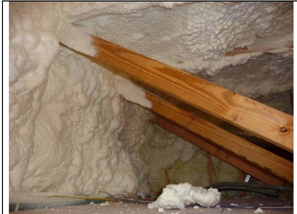
Figure 21 Foam applied to wall and ceiling of the bonus room floor cavity (3' high). (Withers)
