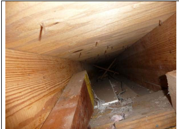
Figure 14 View from soffit vent looking inside towards floor space in area having no batts. (Withers)
