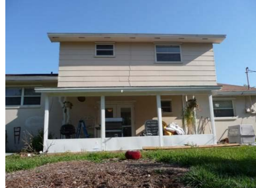
Figure 12 Back of home (facing south) with top story floor space cantilevered and vented over back patio.
