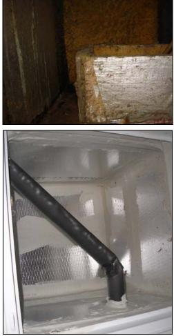
Figure 4 Typical building cavity used as a central return plenum (top) converted to a ducted return sealed with masti (bottom).
