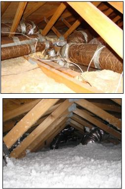
Figure 5 Typical attic insulation preretrofit (top) and post-retrofit (bottom)
