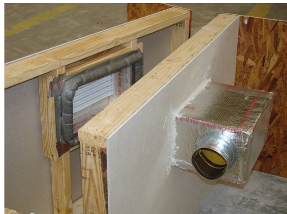
Figure 3 Southern Energy crossover mockup
