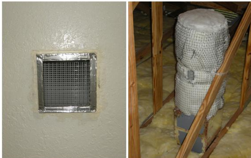
Figure 2. Ceiling penetration for planned leakage (left); attic view of hole that diffuses airflow (right)
