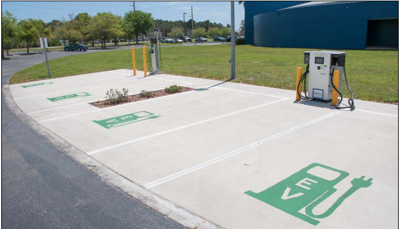
Figure 1. FSEC Public Dual AC Level 2 (left) and DC Fast (right) Charging Stations
