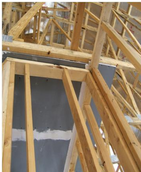
Figure 3. Drywall slipped through \frac{3}{4} -in. space between the top plate of the nonload-bearing interior wall
