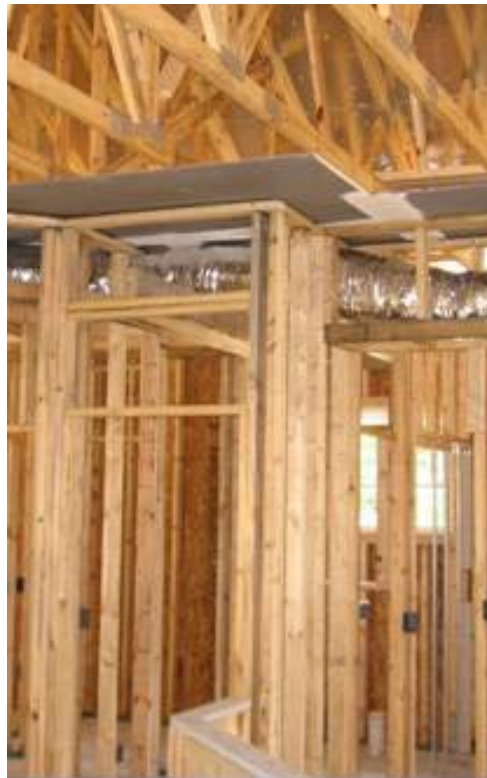
Figure 1. FDC after rough framing
