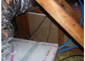
Figure 4-17. Photo shows an area of kneewall missing insulation in an old code home (H59).
