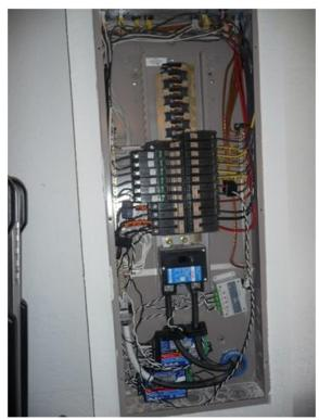
Figure 4-2. Watthode power meters and Hobo data logger energy monitoring system after being installed in an electric panel by a licensed electrician.
