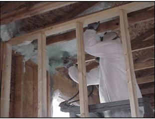
Figure 20. Sealed attic home under construction in Ft. Figure 21. Insulating foam being applied to a 5-inch
