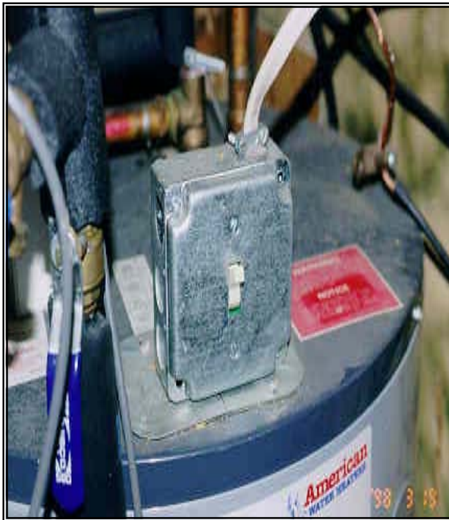
Figure 1.3-13. Electric on/off switch being installed on water heater.
