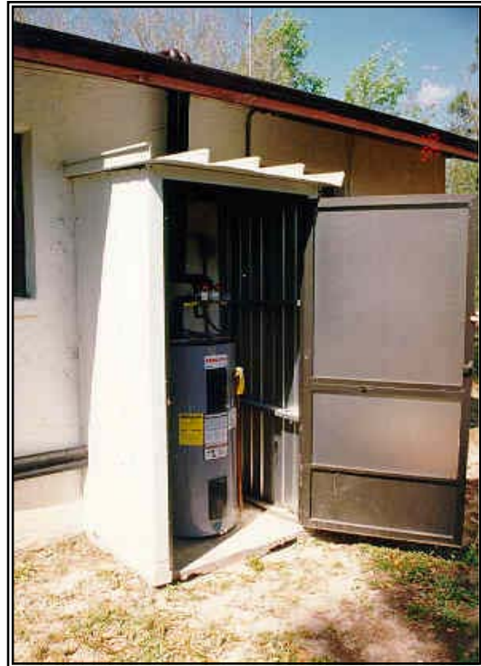
Figure 6.3-20b. Protected water heater and solar components.
