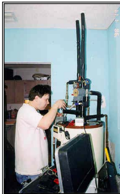
Figure 6.3-3. Working in restricted areas.
