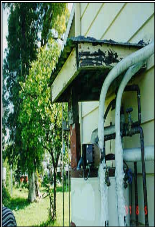
Figure 6.3-20a. Minimal water heater and component protection.
