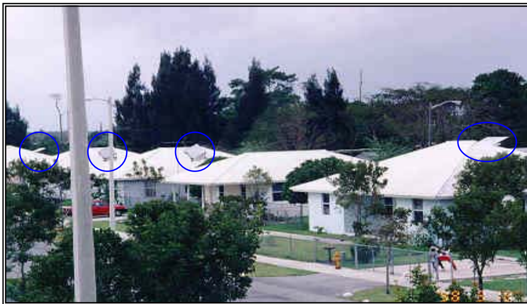
Figure 2.3-5. Low-income residential area in Dade County using SWAP solar systems.
