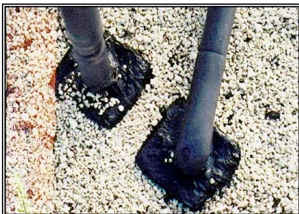
Figure 2.3-1. Pitch pan filled with bitumen.
