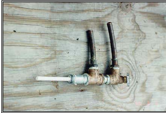
Figure 1.3-9. Tank bottom feed/return valve used in timer controlled systems.
