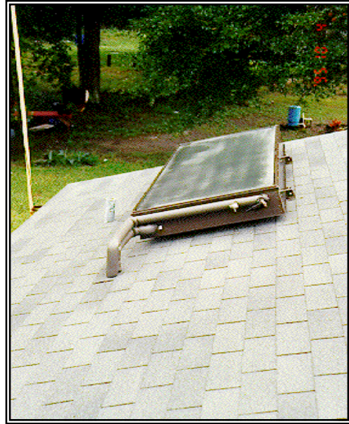
Figure 6.3-9b. Well protected insulation will last many years.
