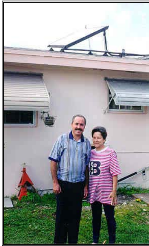
Figure 1.10-1. South Florida system installation at the Matos' residence. The solar system serves both Mr. and Mrs. Matos', as well as their two children. In the summer, they have learned to keep the water heater electricity off and allow the solar system to heat all the water.
