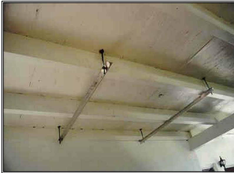
Figure 2.2-2. Spanner mounting of solar collector.
