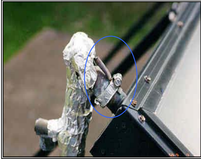
Figure 6.3-13a. Collector sensor secure but not insulated or protected from environmental degradation.
