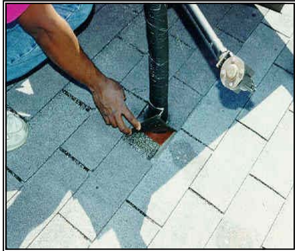
Figure 2.3-4. Ideal roof flashing using copper flashing shown in Figure 2.3-3.
