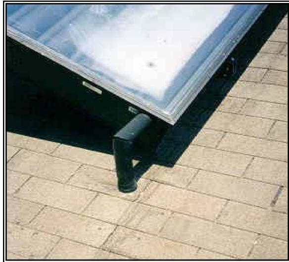
Figure 6.3-11b. Use of 45 degree angle cut and insulation glue provides a positive and aesthetic seal.
