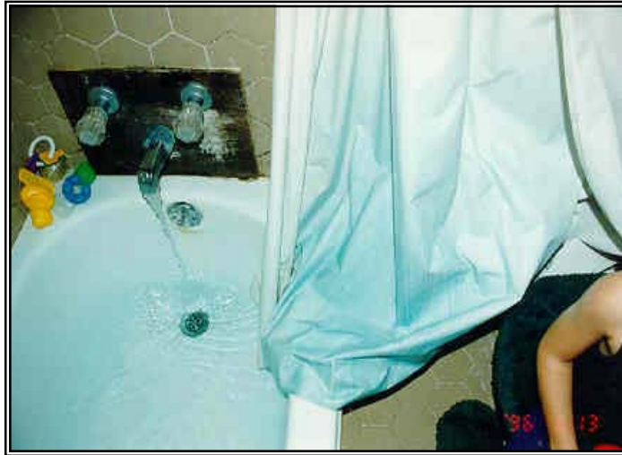
Figure 2.1-6. Blue residue from copper leaching due to very acidic well water.
