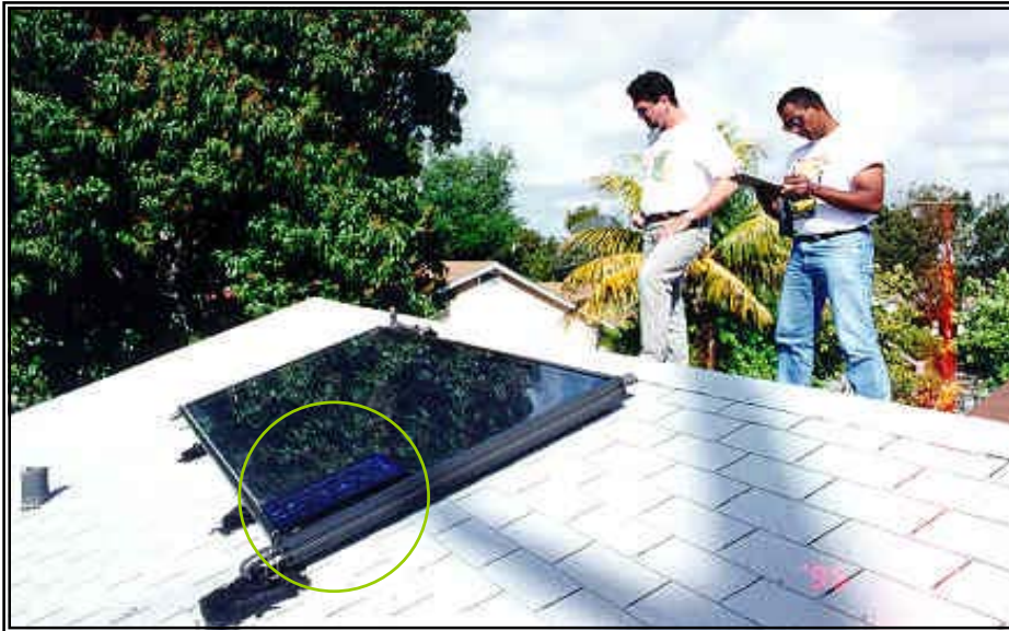
Figure 1.8-1. FSEC staff providing system inspection training for local staff. Lesson learned here - photovoltaic module (on lower right corner of flat-plate collector) is not to be affixed to the face of the flat-plate collector.
