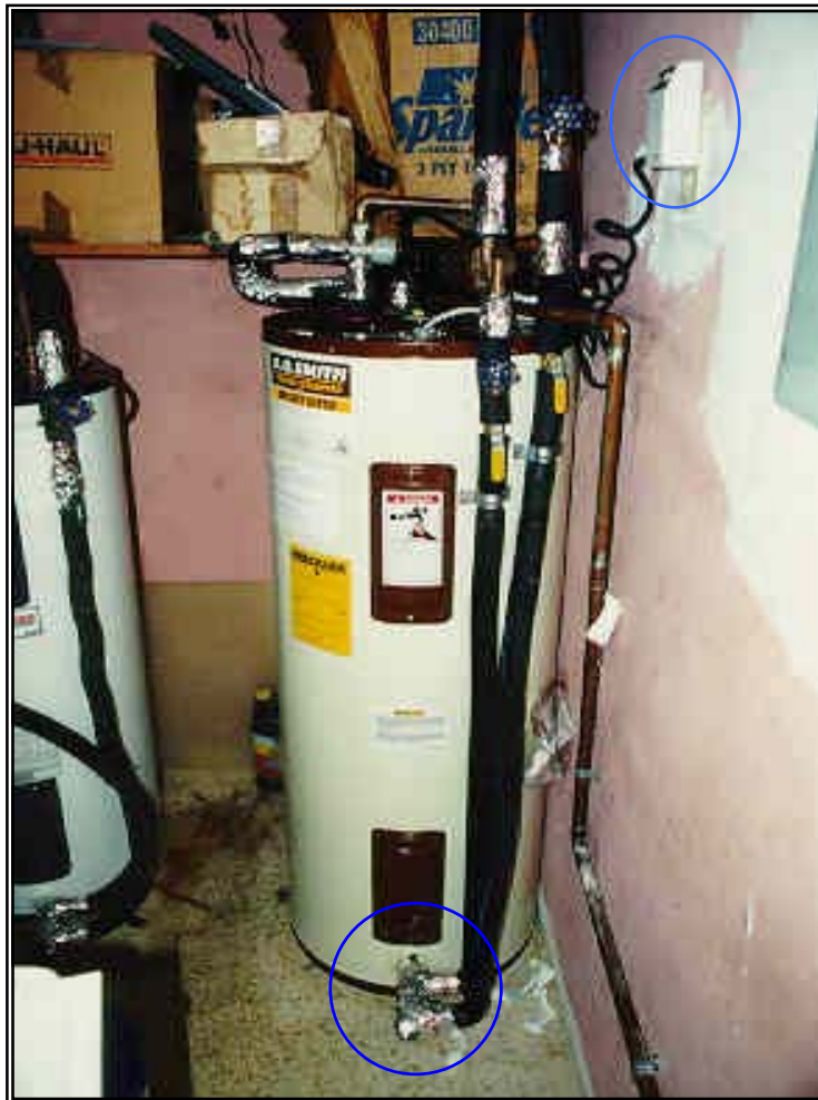
Figure 1.3-10. Tank bottom feed, bottom return valve installed at drain of water heater. Note timer attached to wall at right.
