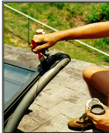
Figure 6.3-8b. Care is taken to make sure that all exposed piping and sensor wires are ultraviolet ray protected.
