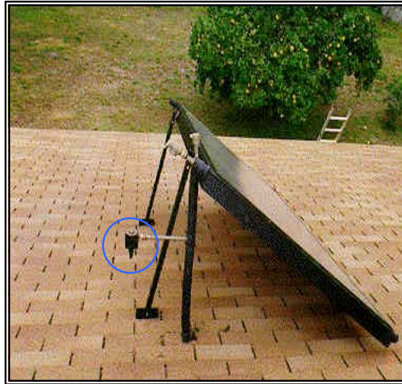
Figure 1.3-8. Freeze valve jutting from collector return line.
