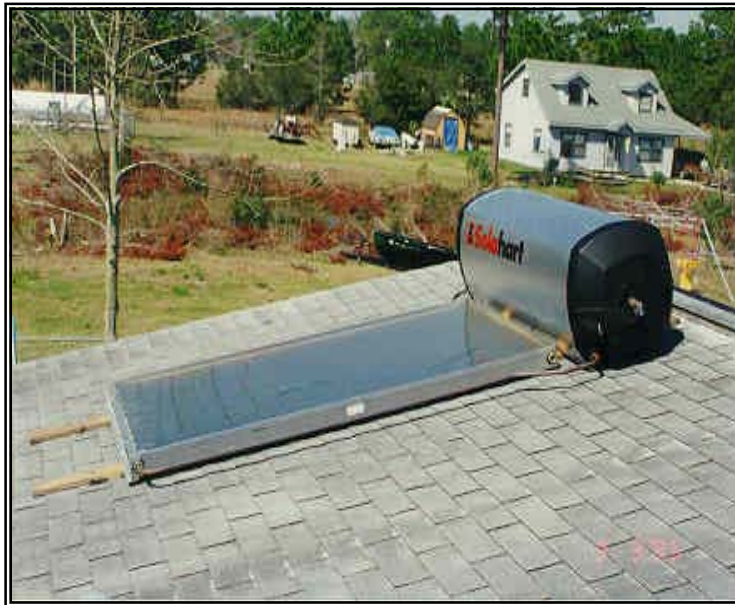
Figure 1.3-3. Thermosiphon system in Central Florida.
