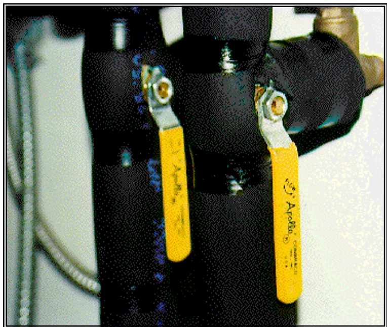
Figure 6.3-16b. Excellent insulation installation.
