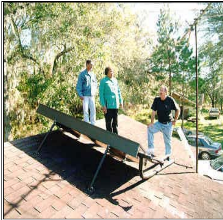
Figure 2.2-1. Brenda Mobley of the Mid Florida Community Services discusses a ICS installation with FSEC's John Harrison and Patrick Robinson.
