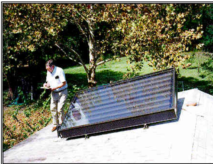
Figure 1.3-1. ICS System in North Florida.
