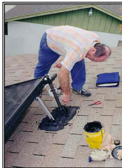
Figure 2.3-2. FSEC's Tom Tiedemann adding bitumen to pitch pan during routine FSEC inspection.
