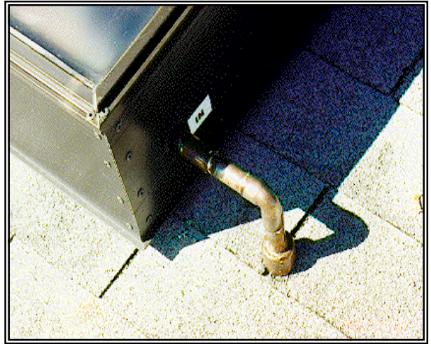
Figure 6.3-7b. Roof flashing is well installed. Insulation is added to cover pipe after copper is soldered.
