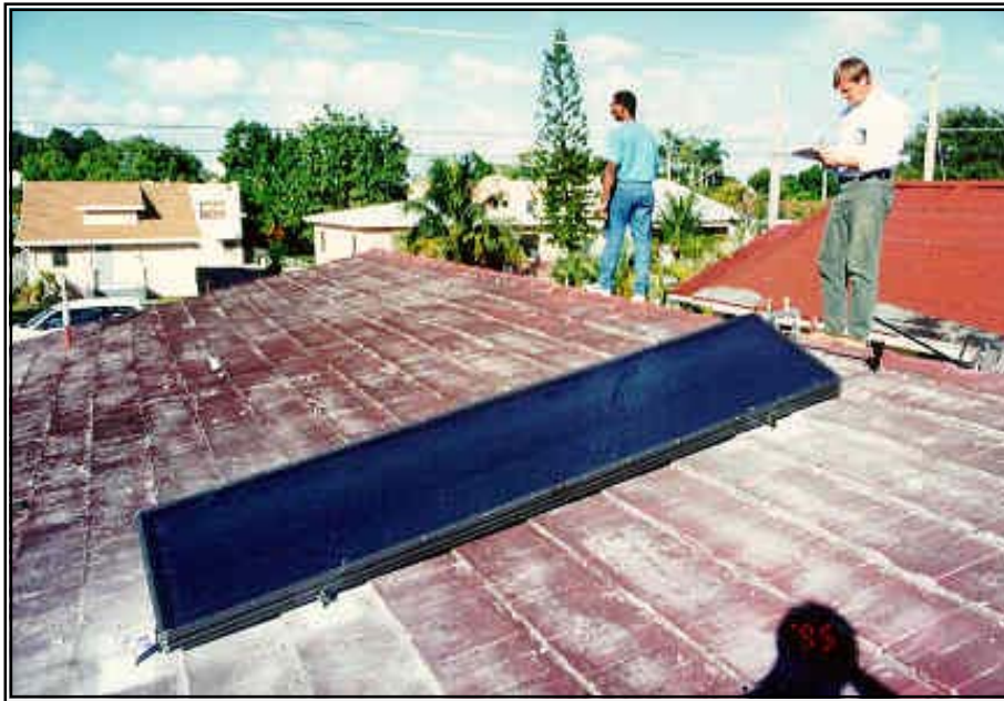
Figure 2.0-1. Twenty-square-foot collector installed on tile roof.
