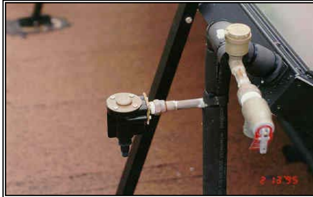
Figure 6.4-1. From left, freeze prevention valve, air vent, and pressure relief valve installed on a flat-plate collector system.
