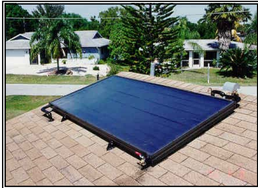
Figure 1.3-4. Flat-plate collector mounted flush to roof.
