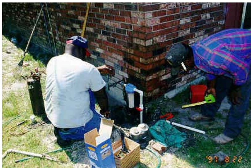
Figure 2.1-5. Whole house filter being installed.
