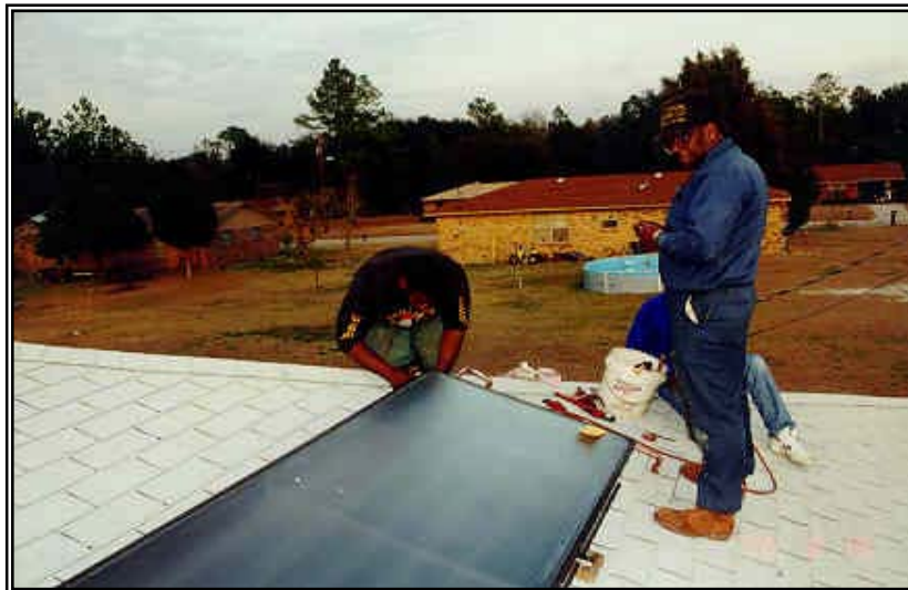
Figure 2.1-3. Local plumber installing ICS system.
