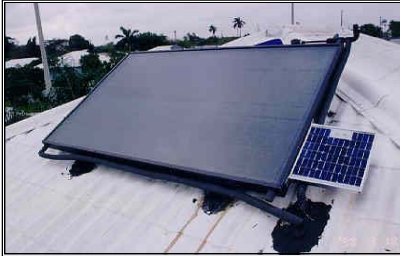
Figure 1.3-11. PV modules installed in plane of flat-plate collector.
