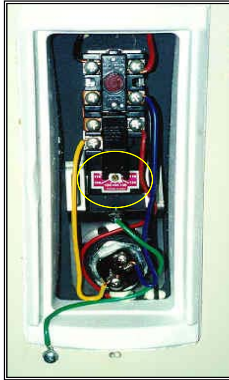
Figure 1.3-15. Water heater thermostat.
