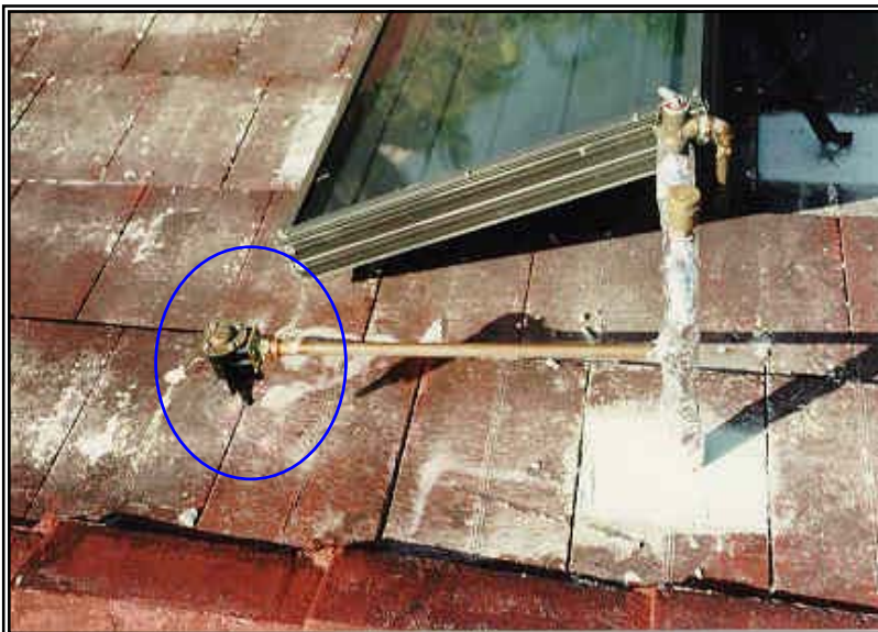
Figure 1.3-12. Freeze valve attached to collector return line. The long non-insulated pipe stub to the freeze valve allows the valve to obtain better ambient temperature readings. It also provides heat release in the summer. Note the foil tape used as protective covering for the pipe insulation.
