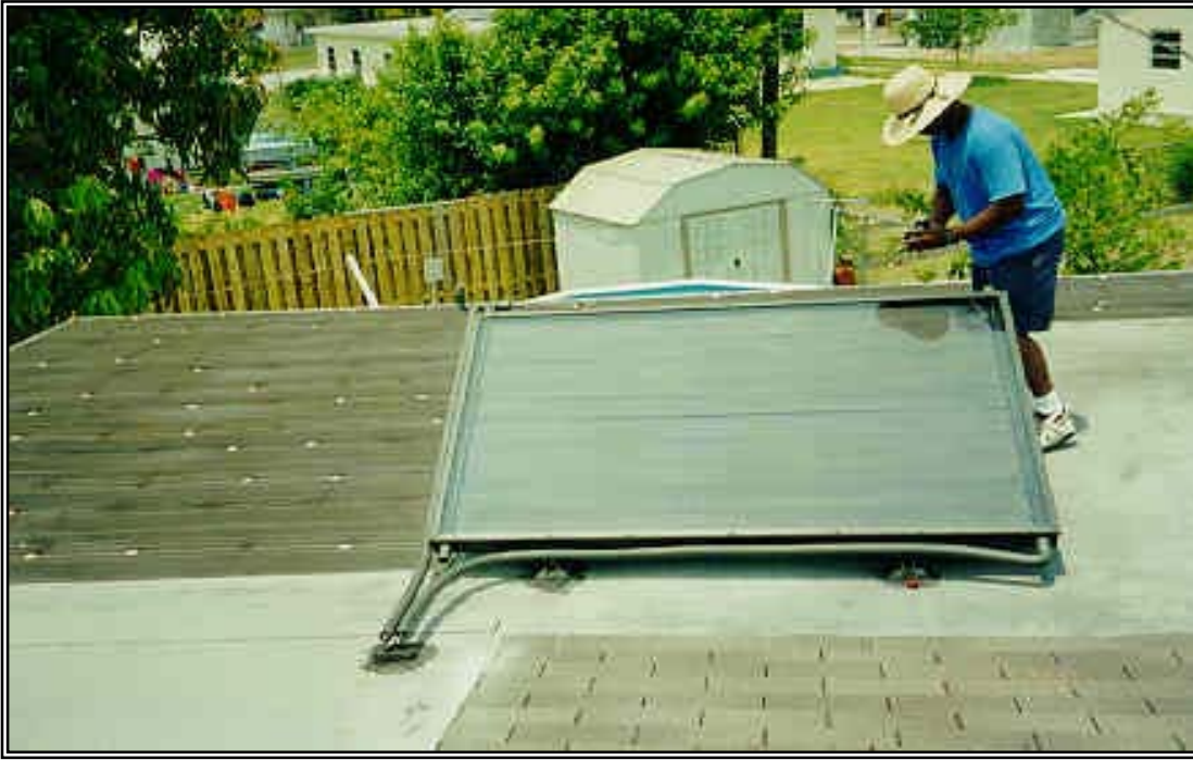
Figure 2.3-6. Twenty-five-square-foot collector installed on Miami site.
