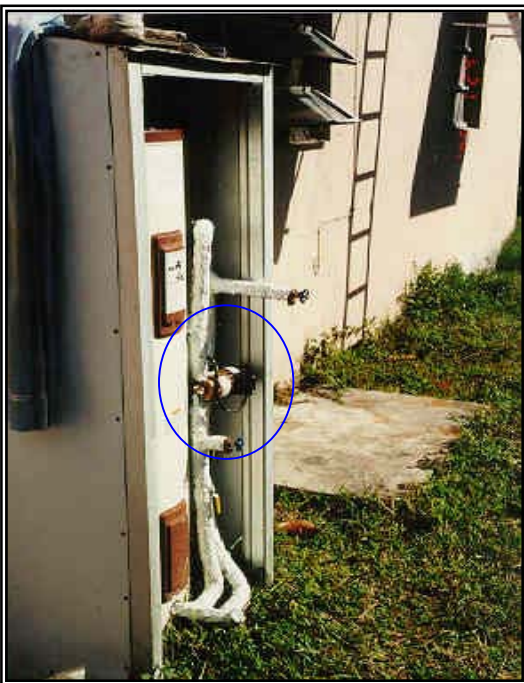
Figure 6.3-18a. Top and sides of water heater protected, but not front. Pump is exposed to elements.
