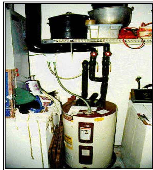
Figure 1.3-2. Water heater and plumbing from ICS system.
