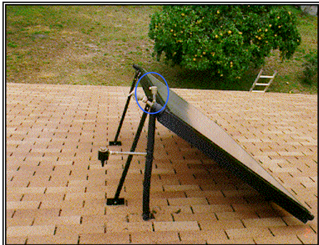
Figure 6.3-12b. Air vent installed in true vertical position.
