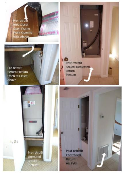
Figure 8. AHU closet with side wall return grille: pre-retrofit (left) and post-retrofit (right)
