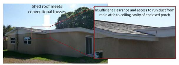
Figure 9. Intersection of shed or flat roof with conventional trusses (left) at enclosed porches creates a very shallow connection (right) to the main attic. Limits room for routing ductwork.
