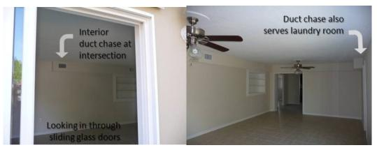
Figure 11. Interior duct chase eliminates need for panned ceiling cavity
