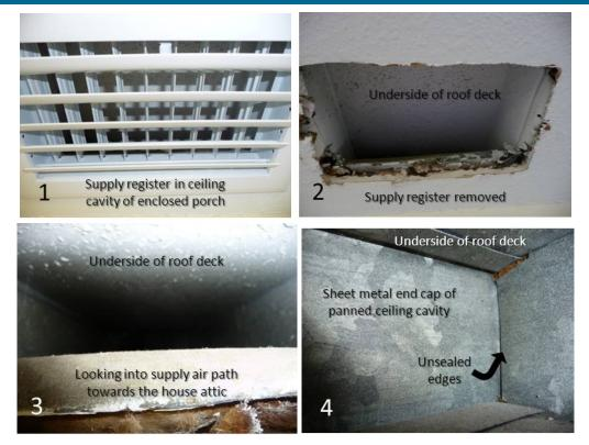
Figure 10. Panned ceiling joist details common to enclosed porches
