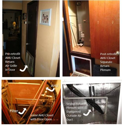
Figure 7. Pre-retrofit AHU closet with no dedicated return (left); post-retrofit with dedicated return and outside air ventilation (right)
