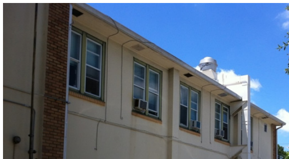
Figure 3. Eaves and vented attic of the Beacon House
