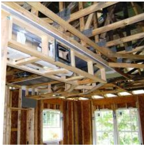
Figure 2: Interior duct system showing roughed in ducts and framing details.
