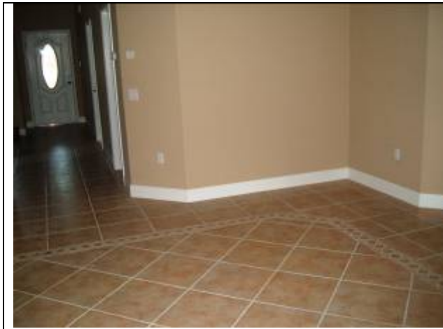
Figure 4. Eighty percent tile floors in the NZEH home improves earth contact cooling.
