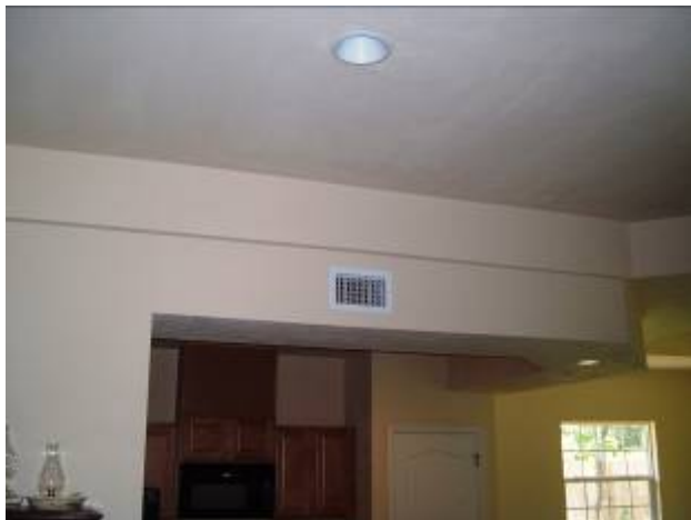
Figure 3. Finished interior duct system passing over kitchen area.
